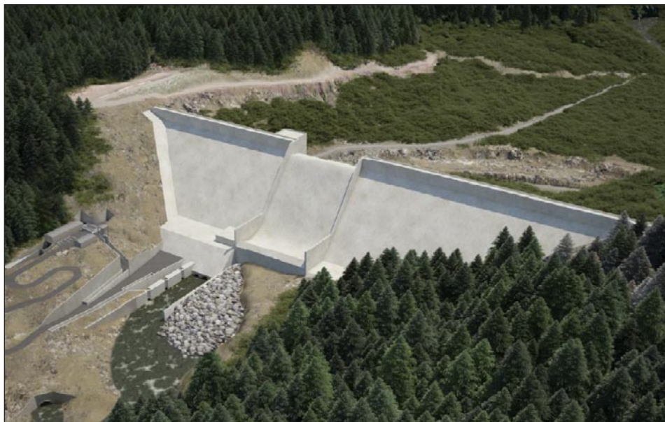
Artist’s rendition of the proposed 250-foot-tall flood control dam on the lower Chehalis River. Photo Courtesy Washington Department of Ecology
